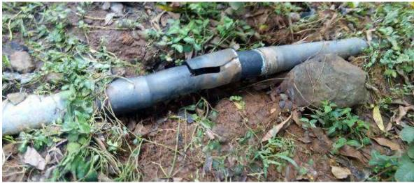
Plate 4.2: A dilapidated water pipeline from the Irate – Nginda scheme which is prone to damages, bursts and leaks in the rough terrain
