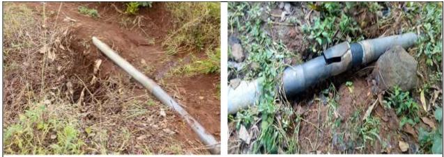
Plate 5.1: Dilapidated Irate Line Exposed Section
