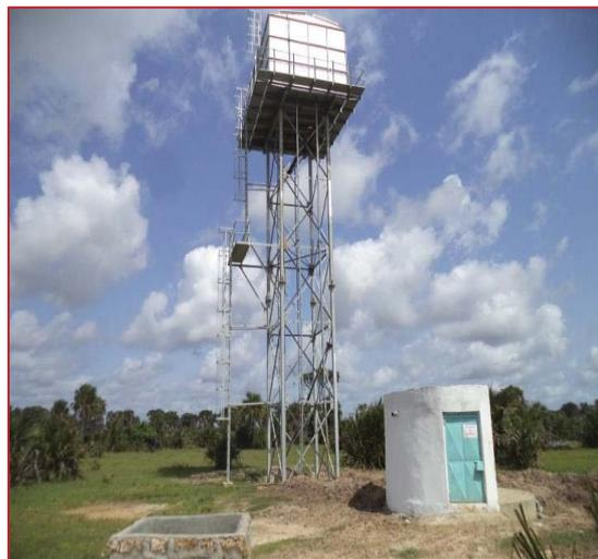
Installation of solar system and completed 60m<sup>3</sup> elevated steel tank on a 15m tower and pump house, Pangani water project, Lamu County
