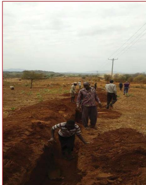
**Preparation of pipeline trench to receive Pipes at Kibunga Kakimiki water project.**
