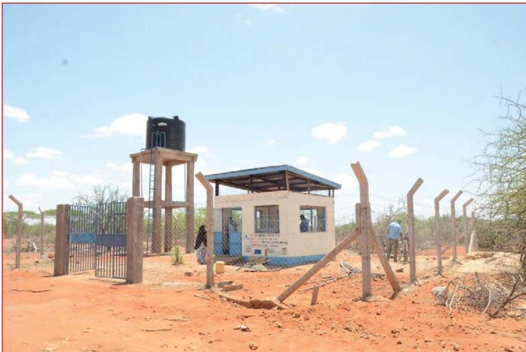
A pump house, platform & fenced borehole site at Shimbrey project, Garissa County
