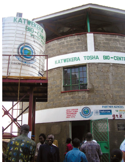
BioCentre facility in Kibera
