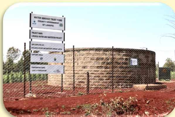
Newly Completed 135m 3 Masonry Tank in Limunga Location under the WSTF Joint 6 Program (J6P)
