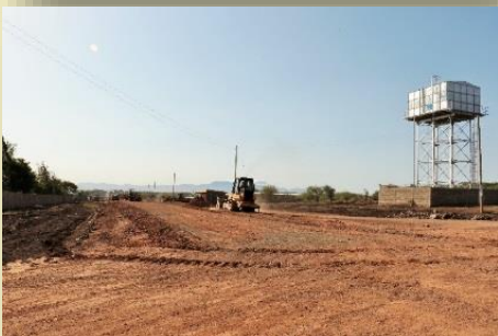
Constructed elevated 165m 3 steel tank along the Isiolo airport Road
