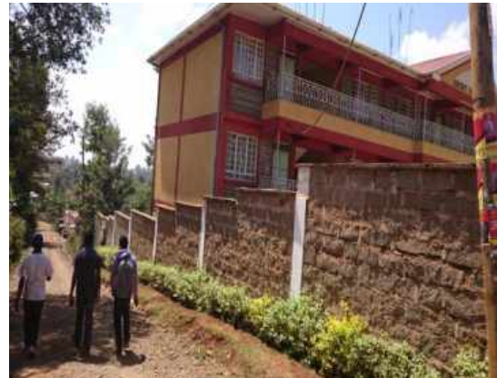
Residential house in Gatende that is set to benefit from the proposed Nyewasco project.
