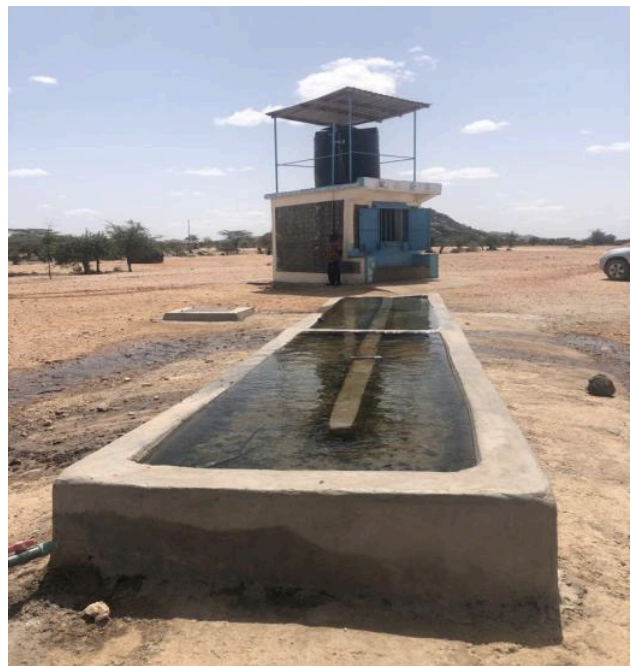
A filled animal watering trough at Lokichar Water Project, Turkana County
