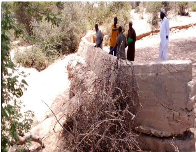
A sand dam at Buriya WRUA, Wajir County
