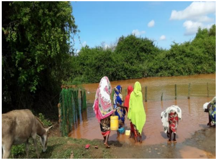
Malkas in River Tana to protect animals and human from the infamous Tana crocodiles
