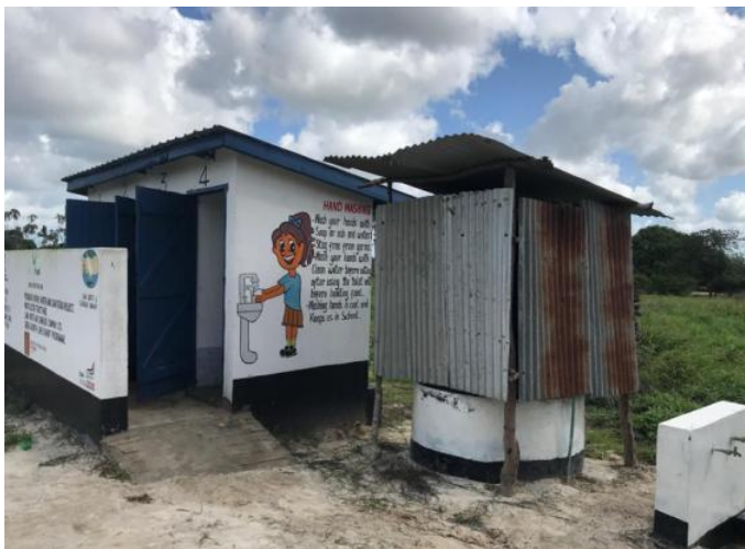
Completed 4-door VIP latrine at Mikinduni primary school with handwashing point and hygiene promotion, Lamu County
