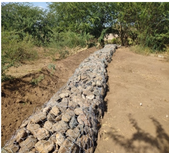
Climate proofing boreholes in Kakuma using gabions
