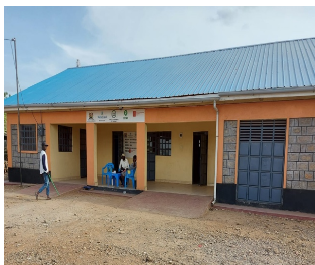
Bio sanitation facility at Kakuma Market
