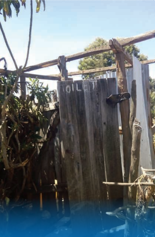
Pit latrines in Maina Village prior to construction of the SafiSan toilets
