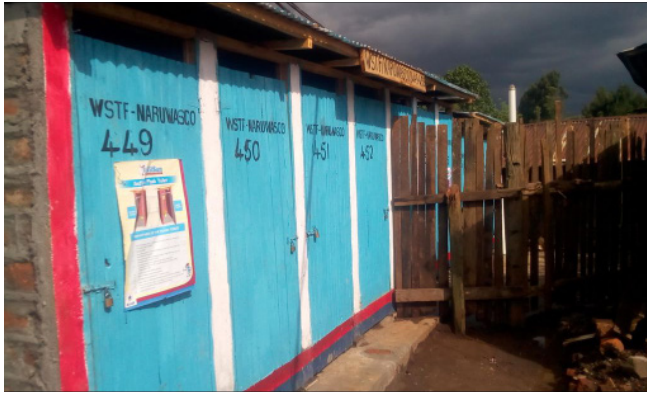
Pour-flush household sanitation, Molo Household Sanitation Project, UBSUP (2015/16), Nakuru
