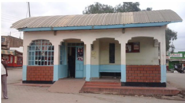
Public Sanitation Facility, Makadara Water Project, UPC Programme (2012/13), Machakos County
