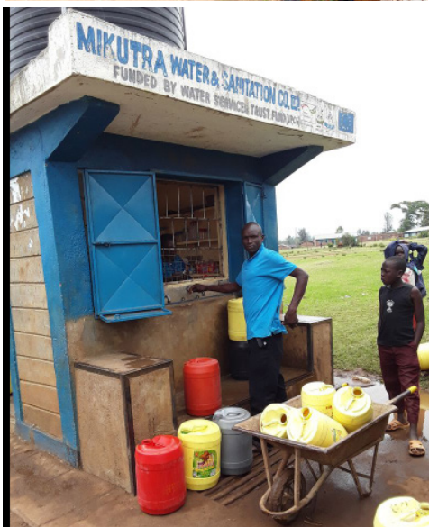
Water kiosk, Awendo Jiwendi Water Project, UPC Program (2014/15), Migori County
