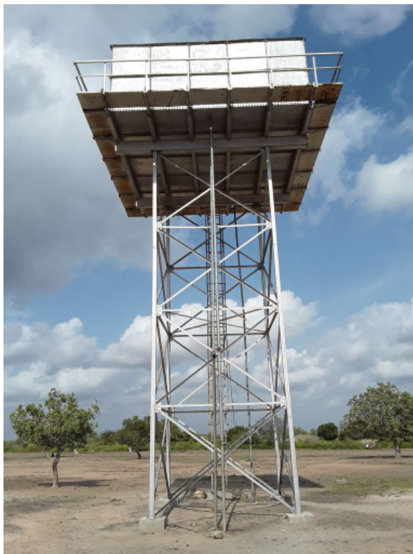
Elevated steel tank, Kotile Community Water Project, MTAP II (2015/16), Garissa County
