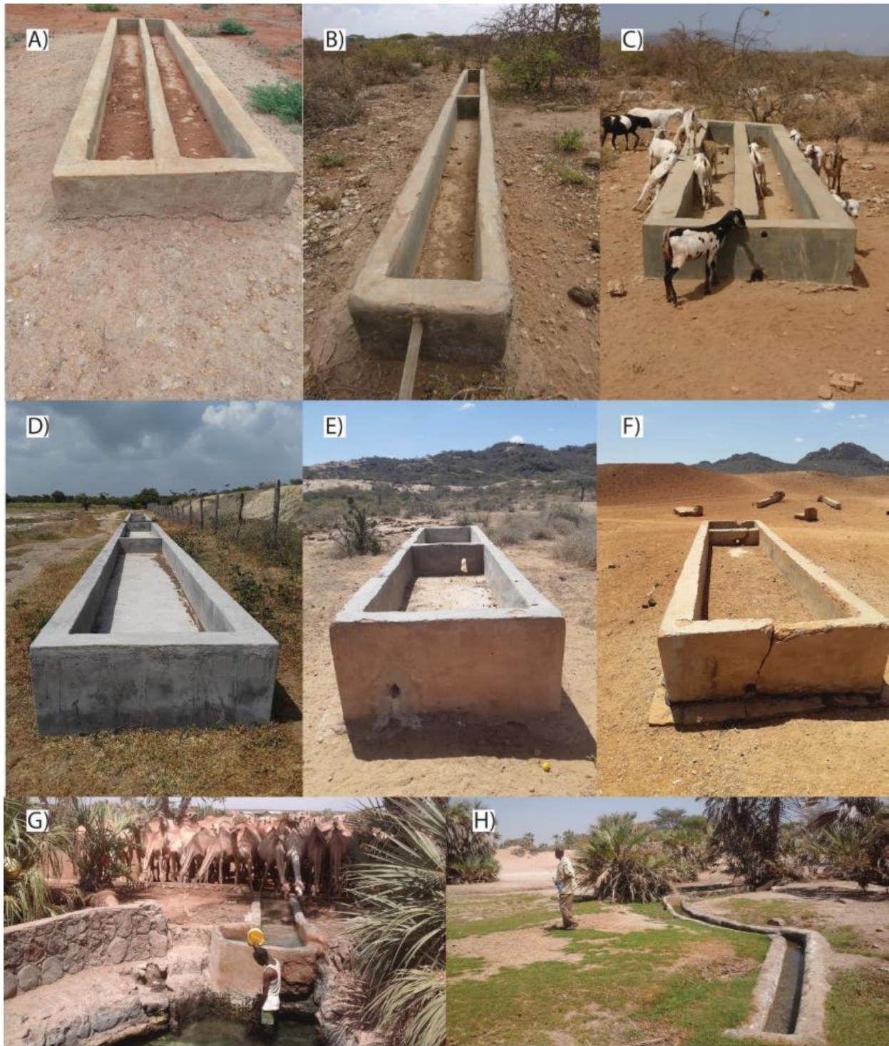
Figure 89. Animal troughs. A) Dhida Community Water project, MTAP II FY 2015/16, Tana River county. B) Gotu, Boji Dera, MTAP II FY 2016/17, Isiolo county; C) Gotu, Boji Dera, MTAP II FY 2016/17, Isiolo county; D) Nairobi Area Community Watsan Project, MTAP II FY 2016/17, Lamu county; E) Ingirir Gumi Gayo water & sanitation project, MTAP II FY 2016/17, Wajir county; F) Buna community water & sanitation project, MTAP II FY 2016/17, Wajir county; G) Galasa Water project, MTAP I FY 2014/15, Marsabit county; H) North Horr Water project, MTAP I FY 2014/15, Marsabit county.
