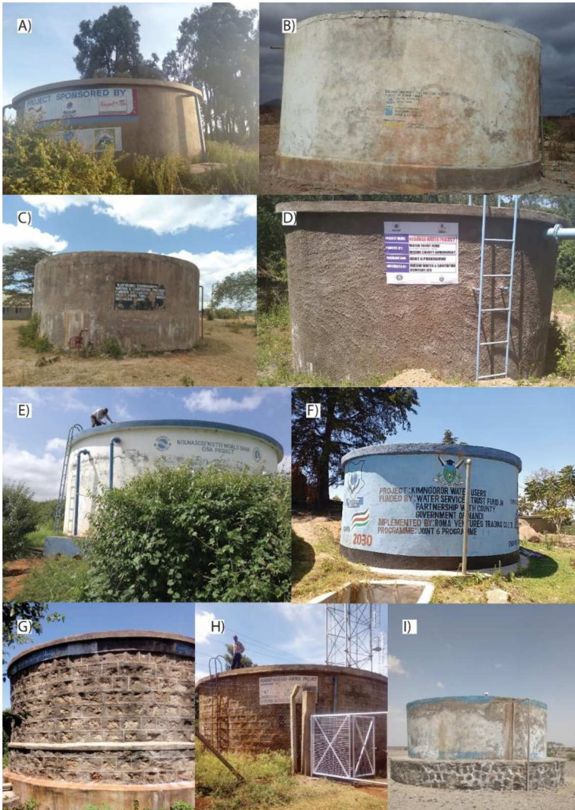
Figure 87. Masonry tanks. A) Timau Water Project, UPC FY 2016/17, Meru county; B) Gotu, Boji Dera, MTAP II FY 2016/17, Isiolo county; C) Kinyagi Water & Sanitation Project, KWSP FY 2013/14, Muranga county; D) Kegonga Water Project, J6P FY 2017/18, Migori county; E) Nol Turesh Water project, OBA FY 2016/17, Makueni county; F) Kimng'oror Water Users association, J6P FY 2017/18, Nandi county; G) Ndula Water & Sanitation Project, CPC FY 2014/15, Kiambu county; H) Riabai And Kihingo Water Project, UPC FY 2013/14, Kiambu county; I) Galasa Water project, MTAP I FY 2014/15, Marsabit county.
