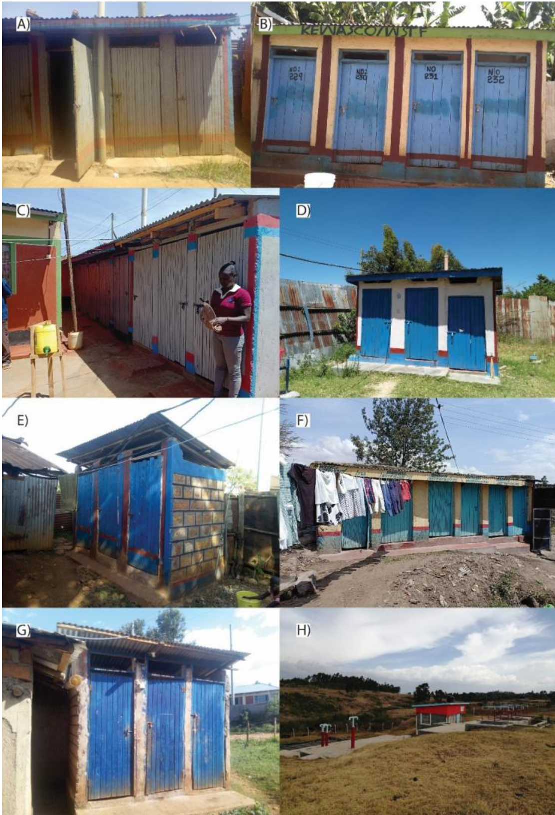
Figure 95. UBSUP Household sanitation. A) Nzoia Kitale Household Sanitation Project Phase I, FY 2015/16, Transnzoia county; B) Kericho Household Sanitation Project Phase II, FY 2017/18, Kericho county; C) Nzoia Kitale Household Sanitation Project Phase II, FY 2015/16, Transnzoia county; D) Machakos Kathemboni Household Sanitation Project Phase II, FY 2017/18, Machakos county; E) Gusii Household Sanitation Project, FY 2015/16, Kisii county; F) Nakuru Household Sanitation Project Phase II, FY 2017/18, Nakuru county; G) Gusii Household Sanitation Project, FY 2015/16, Kisii county; H) DTF, Ol Kalou Household Sanitation Project, FY 2017/18, Nyandarua county.
