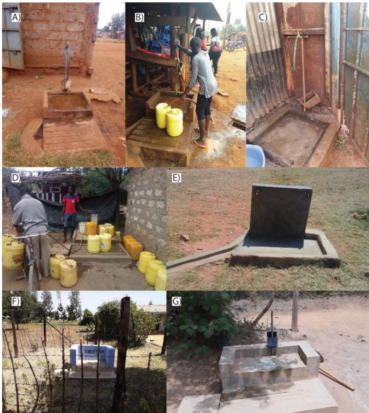
Figure 90. Yard taps. A) Nyagacho, Satellite & Chebocho Water Project, UPC FY 2016/17, Kericho county; B) Indian Burzar Water Project; UPC FY 2014/15, Kiambu county; C) Rockline Water Project, UPC FY 2014/15, Kiambu county; D) Malindi Informal Settlements Water Project, UPC FY 2013/14, Kilifi county; E) Luisukut Water Project, J6P FY 2017/18, Laikipia county; F) Sirimon Self Help Water Project, J6P FY 2017/18, Laikipia county; G) Nyasanda Ugunja Water Project, UPC FY 2016/17, Siaya county.
