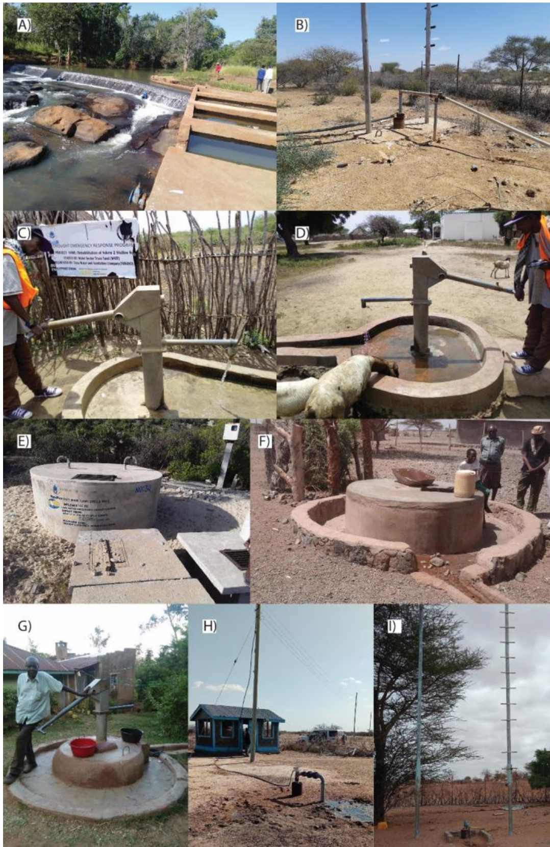
Figure 92. Intakes. A) River intake, Kathwana Water Project, J6P FY 2017/18, Tharaka Nithi county. B) Borehole, Boji Garas Community water & sanitation project, MTAP II FY 2016/17, Wajir county. C)-D) Hand dug well, Rehabilitation of Ndura(1), Ndura(2), Handaraku and Marava shallow wells, DERP FY 2017/18, Tana River county. E) Lamu Dunes Well 2no., DERP FY 2017/18, Lamu county. F) Rehabilitated shallow well, Galasa Water project. MTAP I FY 2014/15, Marsabit county; G) Hand dug well, Jekpoyai Water Project, CPC FY 2013/14, Vihiga county. H) Skanska Boreholes, DERP FY 2017/18, Garissa county. I) Bahuri Boreholes, DERP FY 2017/18, Garissa county.
