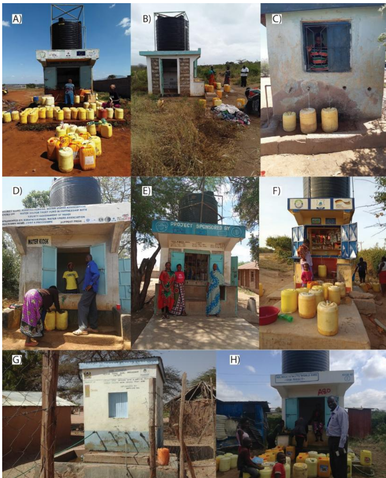
Figure 88. Water kiosks. A) Mwana-Wikio Water Project, UPC FY 2013/14, Kiambu county; B) Taru Gatsakuleni Water Project, J6P FY 2017/18, Kwale county; C) Boji Garas Community water & sanitation project, MTAP II FY 2016/17, Wajir county; D) Kimatkei/Kipkoil Water project, J6P FY 2017/18, Nandi county; E) Kibuyu-Mikunduni Water Project, UPC FY 2013/14, Tana River county; F) Siakago Township Water Project, UPC FY 2013/14, Embu county; G) North Horr Water project, MTAP I FY 2014/15, Marsabit county; H) Nol Turesh water project, OBA FY 2016/17, Makueni county.
