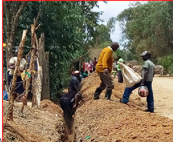
Community doing 7 km trench at Sipili Water Project.
