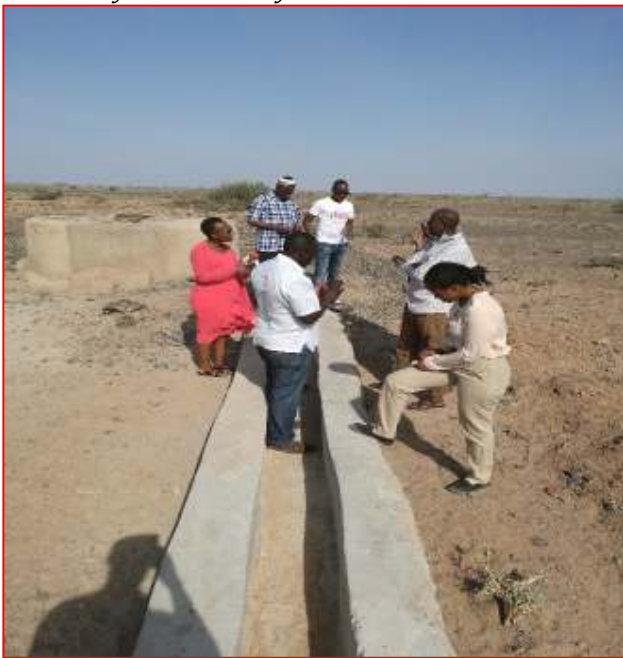
Water trough for Camels – North Horr WRUA
