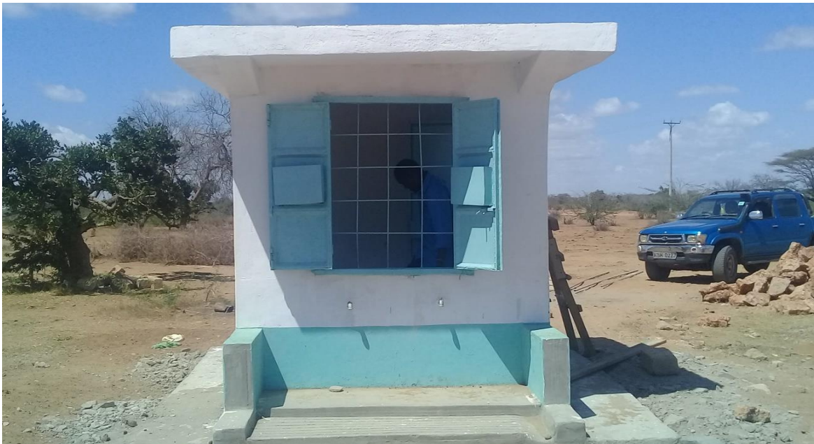
FIGURE 8 PARTIALLY COMPLETED WATER KIOSK AT KORAKORA WATER PROJECT, GARISSA COUNTY
