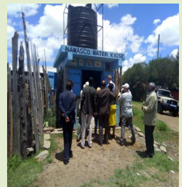
Activated NAWASCO water kiosk at Katheri Centre
