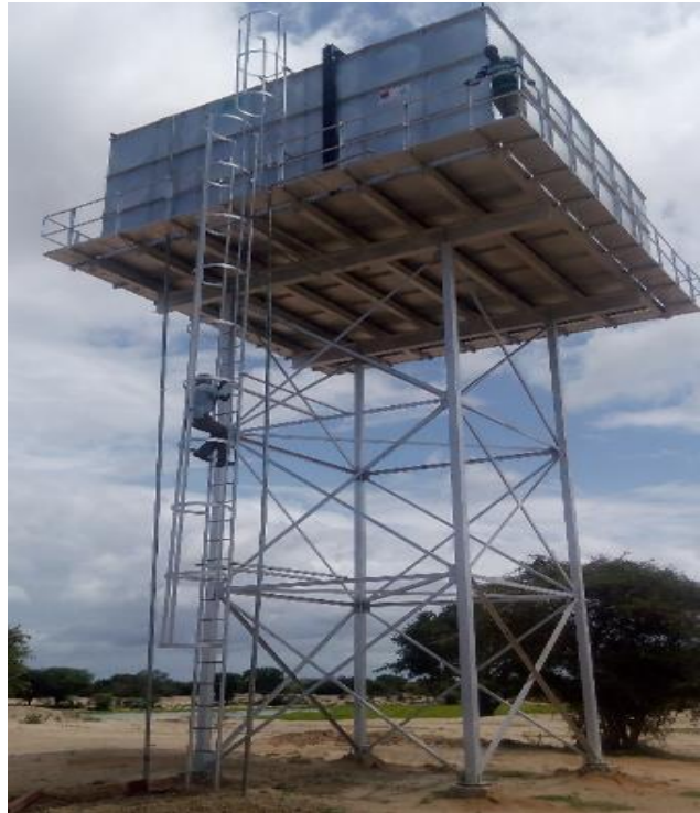
elevated steel tank 150m 3
