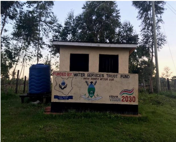
Public Sanitation Facility constructed by Kobujoi Water Project at Kshogon Primary School, Nandi County
