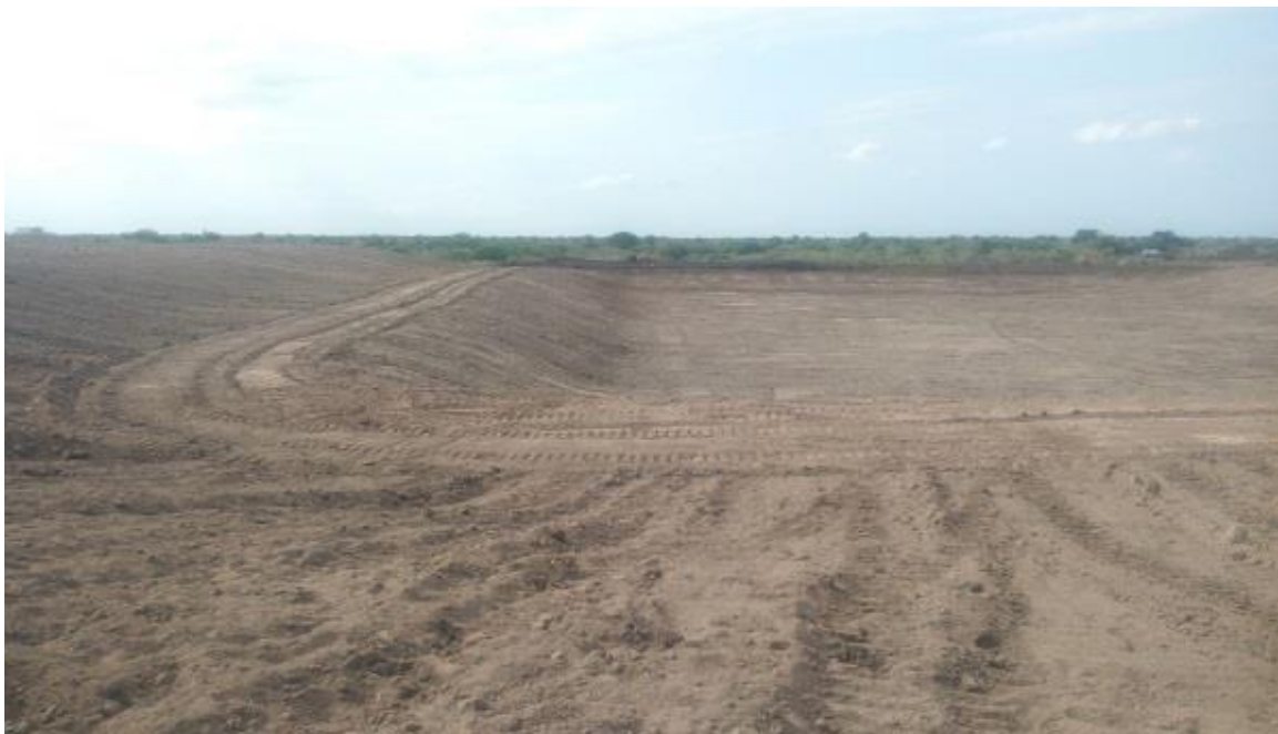
Newly constructed water pan at Gababa water project, Garissa County
