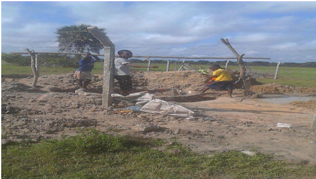
Construction of a shallow well at Mkunumbi, Lamu County
