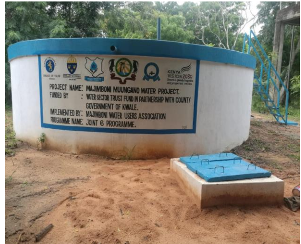
Masonry Water Tank done by Majimboni Muungano Water Project, Kwale County
