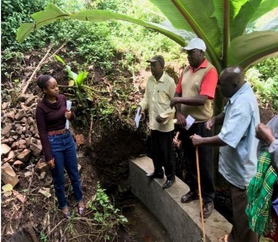
Spring protection construction ongoing by Mbogo WRUA, Nandi County
