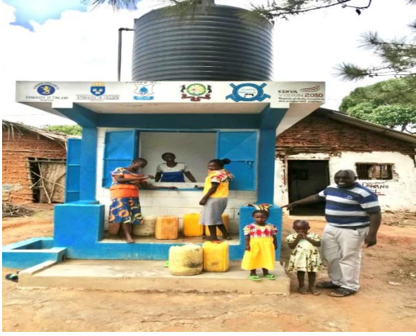
Water Kiosk Constructed by Majimboni Muungano Water Project, Kwale County
