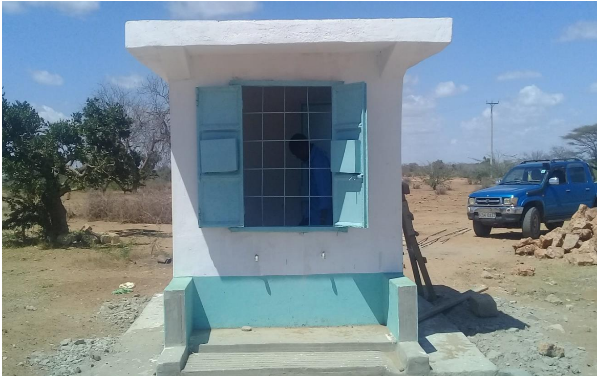
Partially completed water kiosk at Korakora water project, Garissa County
