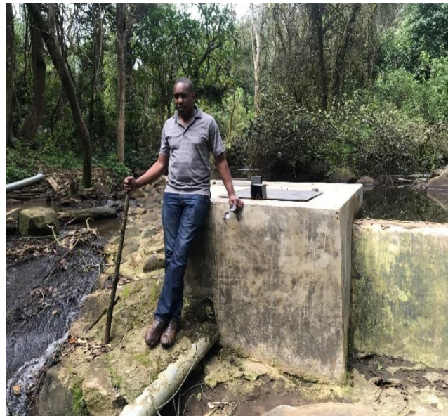
Common Intake constructed at R. Kobujoi, by Kobujoi Water Project
