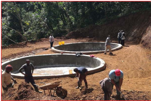
Gatare CFA fishpond installation for trout fish farming ongoing- Murang'a County
