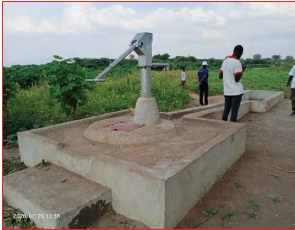
Completed shallow well
