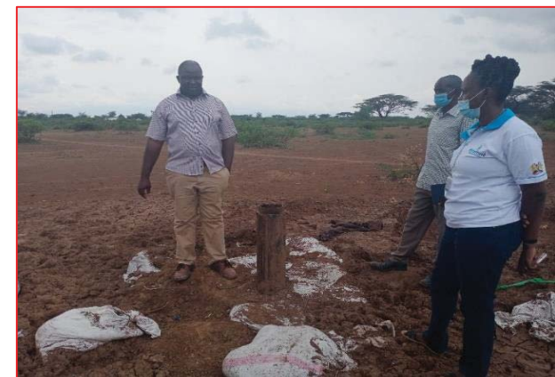
Drilled borehole by oxfam at Nakuangat
