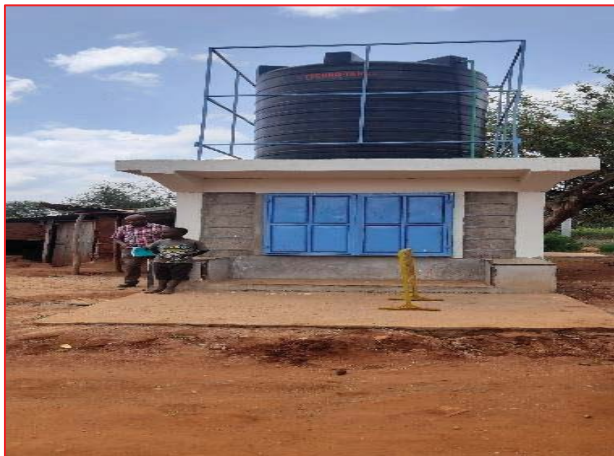
Constructed water kiosk in Kibunga Kakimiki water project and one of the first connections for Solio Settlement Scheme water project.
