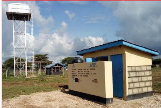
Elevated Steel tank and 2 door VIP latrine at Ngalabilabia Borehole, Isiolo County
