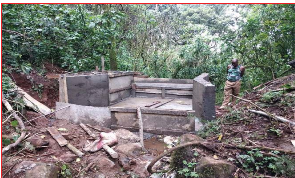
Ongoing construction of an intake for Kimatkei Kipkoil water project.
