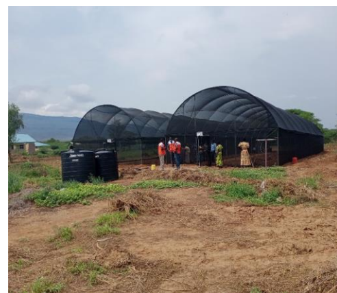
Shade nets (30mx8m) installed at Lokichoggio for horticultural farming
