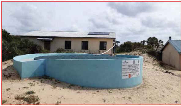
The completed 100m3 underground water tank equipped with submersible pump at Bright Girls Secondary School
