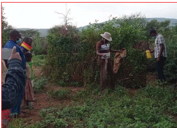
Household latrines constructed as a result of CLTS support
