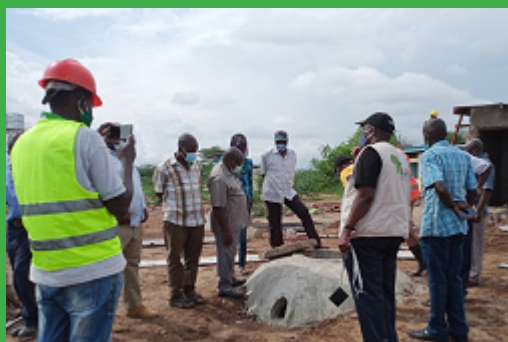
Stakeholders inspecting a bio sanitation dome installation project
