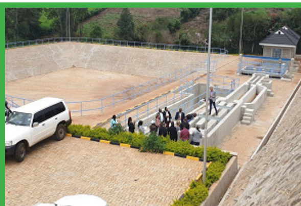
Inspecting a Water Treatment Facility
