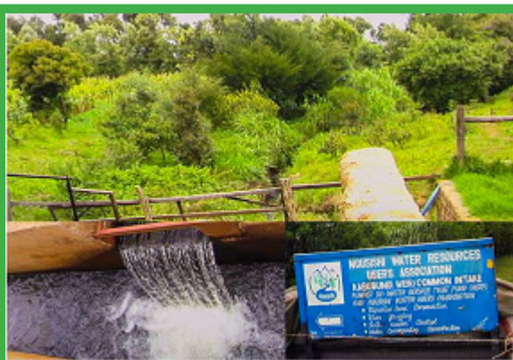
One of the many WRUAs supported
