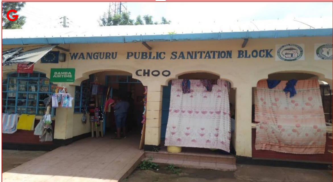
Figure 84: Public Sanitation Facilities (PSFs).
