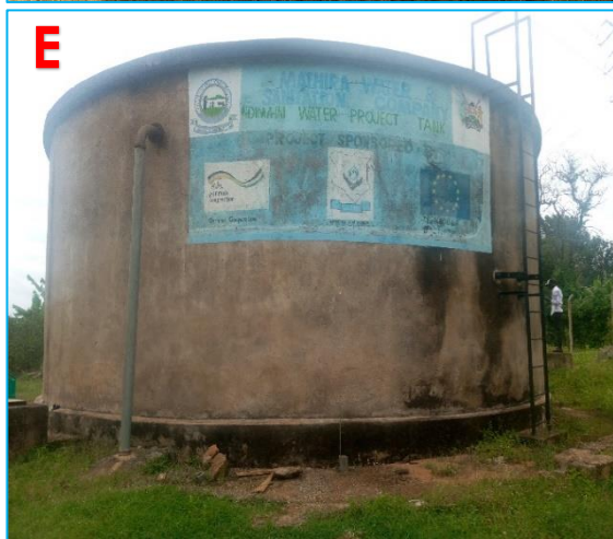
Figure 77: Masonry tanks; various locations
