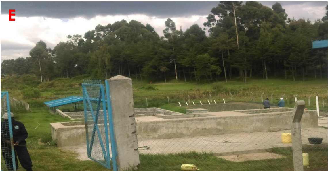
Figure 85: De-centralized Treatment Facilities
