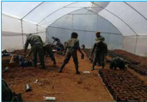
Zaina CFA model greenhouse establishment Nyeri County
