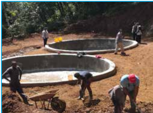
Gatare CFA fishpond installation for trout fish farming ongoing- Murang'a County
