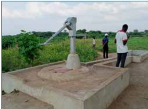
Completed shallow well
