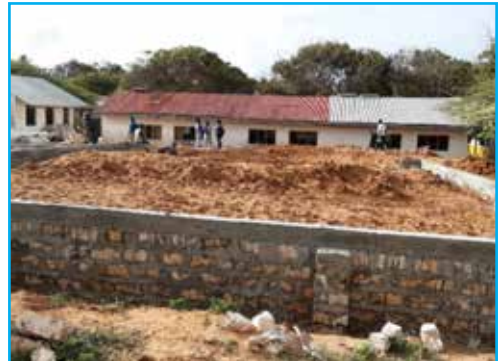
Kiunga Conservancy djabia under construction
