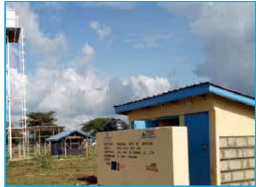
Elevated Steel tank and a two-door VIP latrine at Ngalabilabia Borehole, Isiolo County
