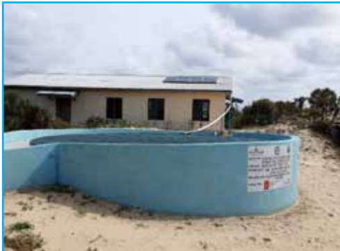
The completed 100m 3 underground water tank equipped with submersible pump at Bright Girls Secondary School
