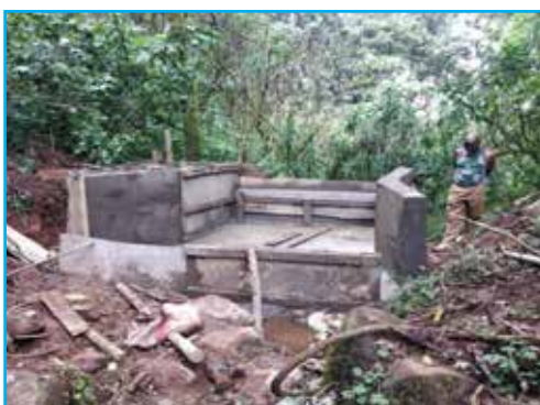
Ongoing construction of an intake for Kimatkei Kipkoil water project
