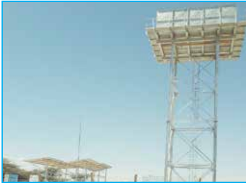
Elevated Steel tank and a two-door VIP latrine at Ngalabilabia Borehole, Isiolo County
