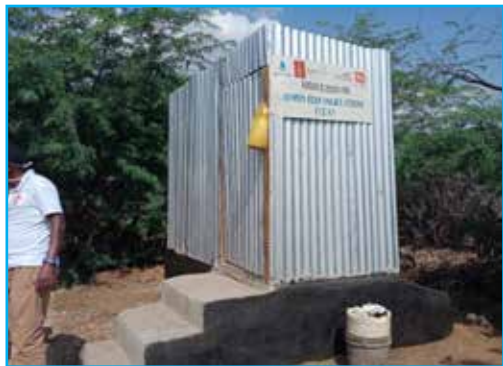
UDDT latrine constructed in kakuma refugee camp
