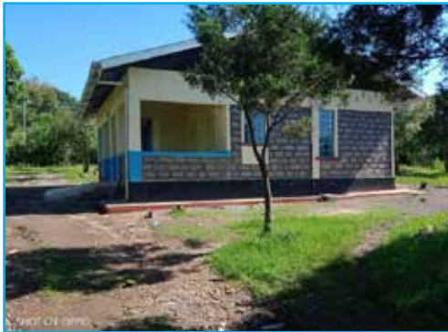
Completed Kilgoris Public Sanitation Facility
