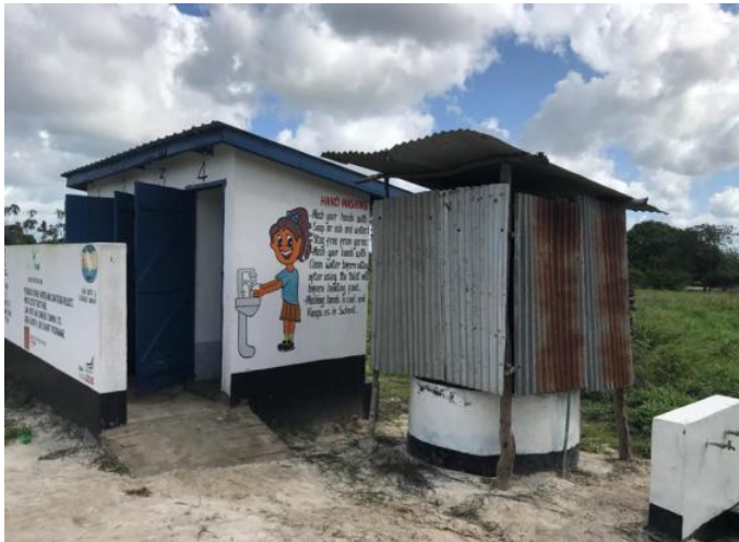
Completed 4-door VIP latrine at Mikinduni primary school with handwashing point and hygiene promotion, Lamu County
