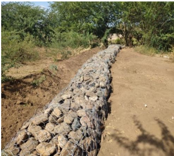
Climate proofing boreholes in Kakuma using gabions
