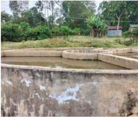
Rongo Riosiri Water Project in Migori
