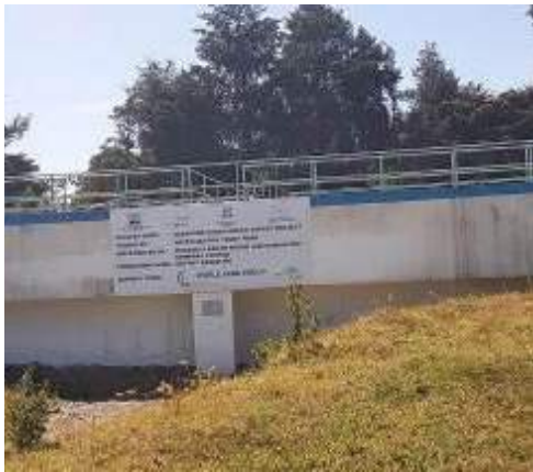
Murang'a South water extension subproject phase II in Muranga
