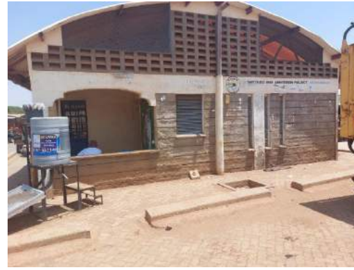
Bus Park Sanitation Project in Taita Taveta
