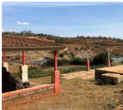
Households Sanitation Project in Machakos
