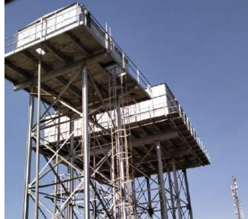
Wanguru Water Supply project in Kirinyaga
