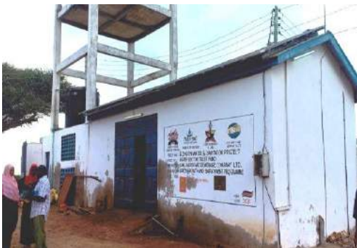
Kizingitini Water and Sanitation Project in Lamu
