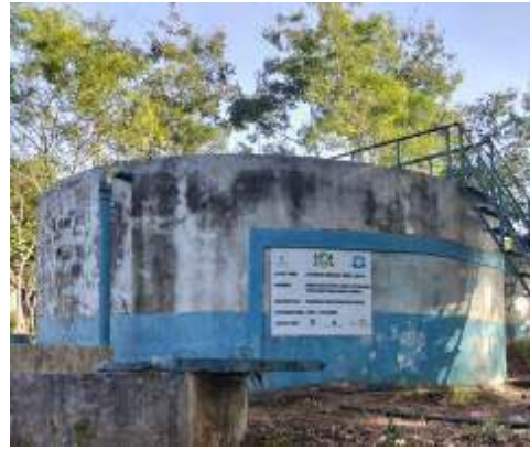
Majimboni Muungano Water Project in Kwale
