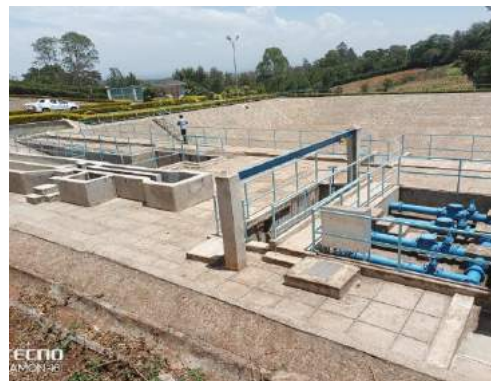
Sewer Extension Subproject in Nyeri
