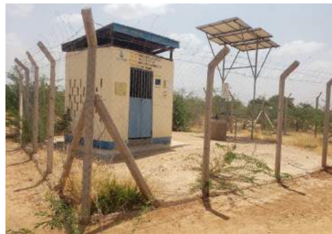
Maramtu B Water Project in Tana River
