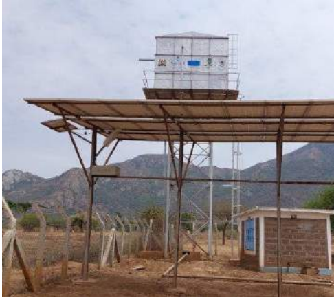
Nyangoro Maktau Water Project in Taita Taveta
