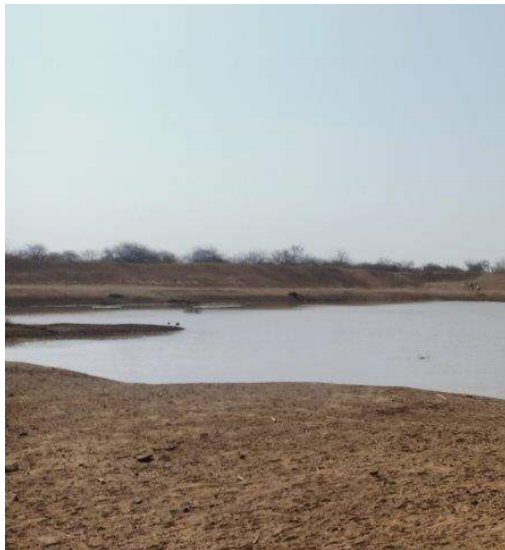
Adadi Jule Water and Sanitation Project in Wajir
