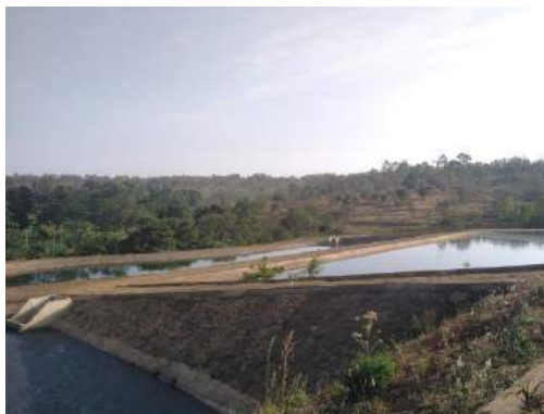
Sewer Extension Subproject in Embu
