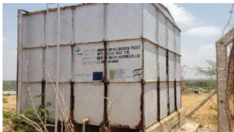
Maramtu B water Project in Tana River
