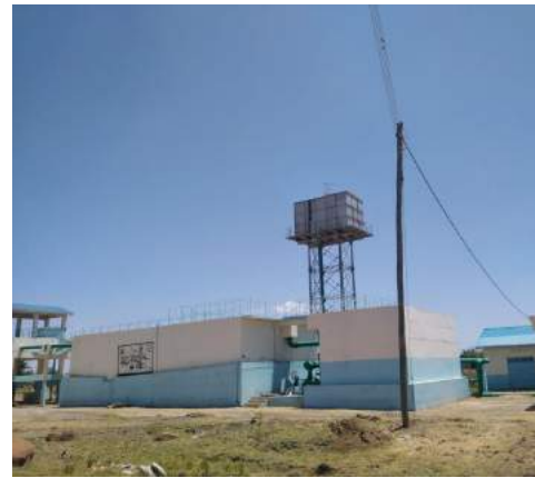
Kathwana Water Project in Tharaka Nithi
