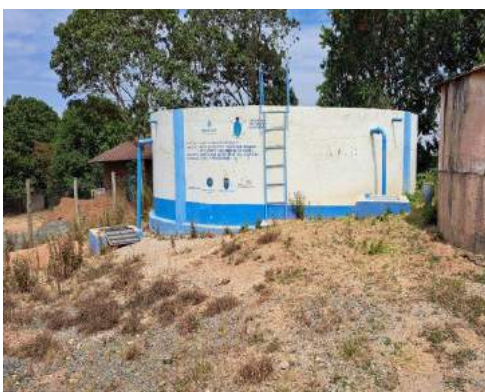
Cheptil water project in Nandi
