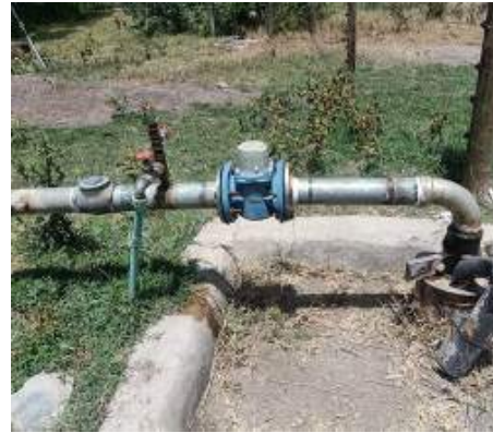
Naivasha water extension subproject in Nakuru
