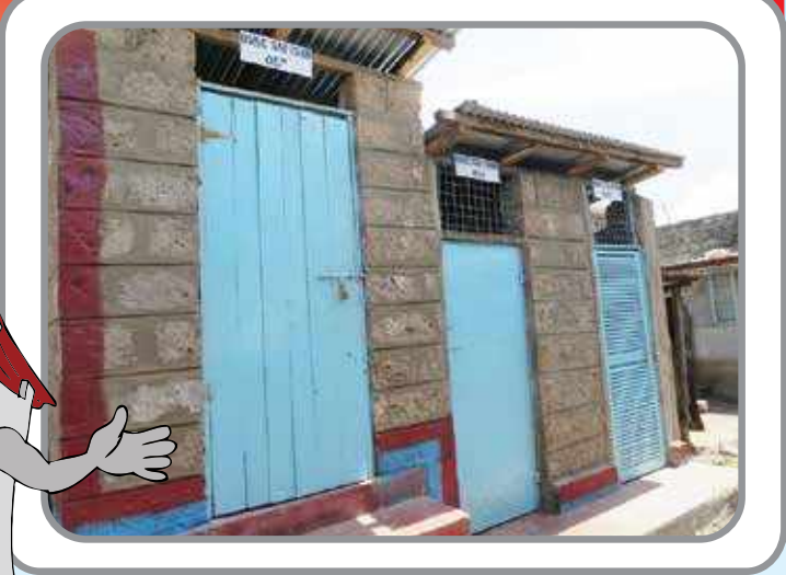
TOILET "A" AFTER REHABILITATION
