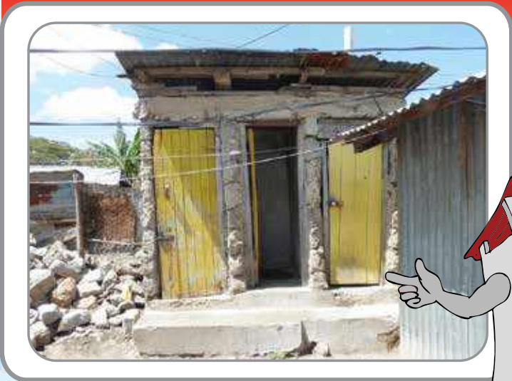
TOILET "B" BEFORE REHABILITATION
