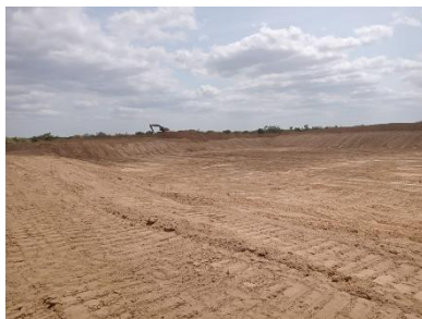
Ongoing Construction of a Water pan in Wenje, Tana River County.
