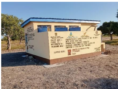
VIP latrine at Hara primary school Garissa County.
