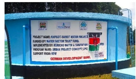
Constructed 150m 3 masonry tank under Kapsoit-Sosiota Water project
