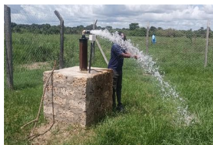
Pumping at Baomo borehole – 28m3/hr in Tana River County
