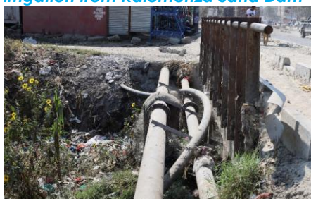
A section of the 2km Pipeline extension in Mavoko town
