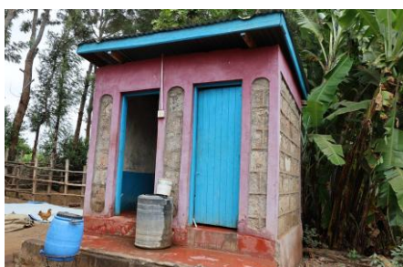
Two-Door Pour-Flush Household VIP Toilets
