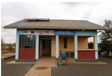
Kabati Public Sanitation Facility in Kitui County
