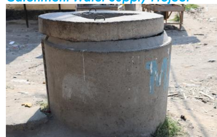
Valve chamber at Kwa Mang'eli in Mavoko Town
