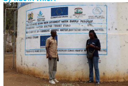
50m 3 Concrete tank at Kyuso Rock Catchment Water Supply Project
