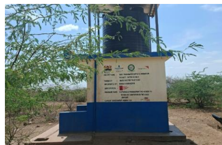
Right: A Water Kiosk in Napopongoit area at Tado Farm Water Supply and Irrigation Project
